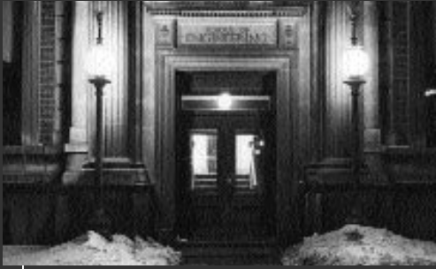
The former School of Engineering in 1948, now Mathematics Hall.
