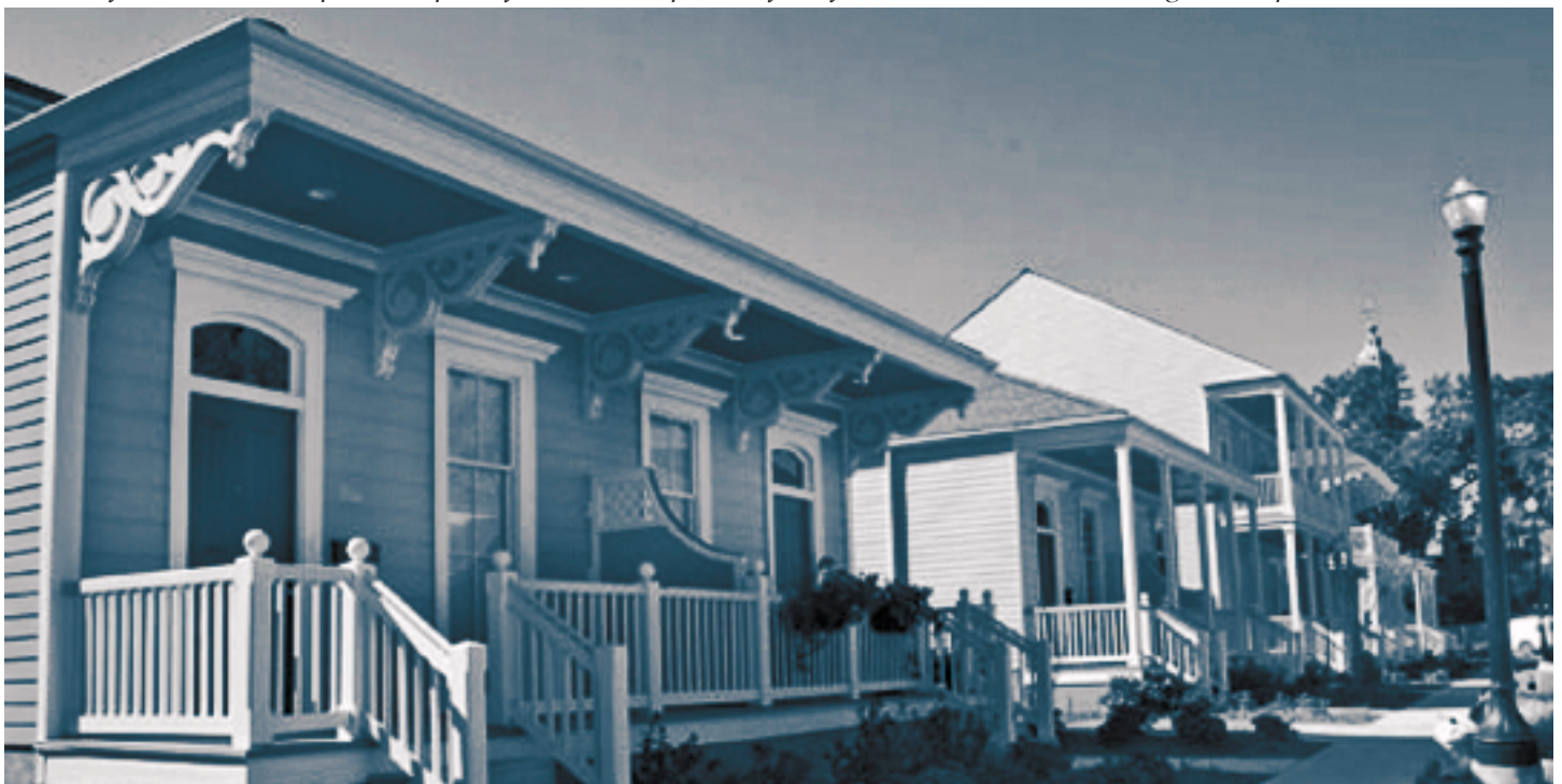
Phase I of River Garden opened as part of the redevelopment of the former St. Thomas Housing Development in District B.
