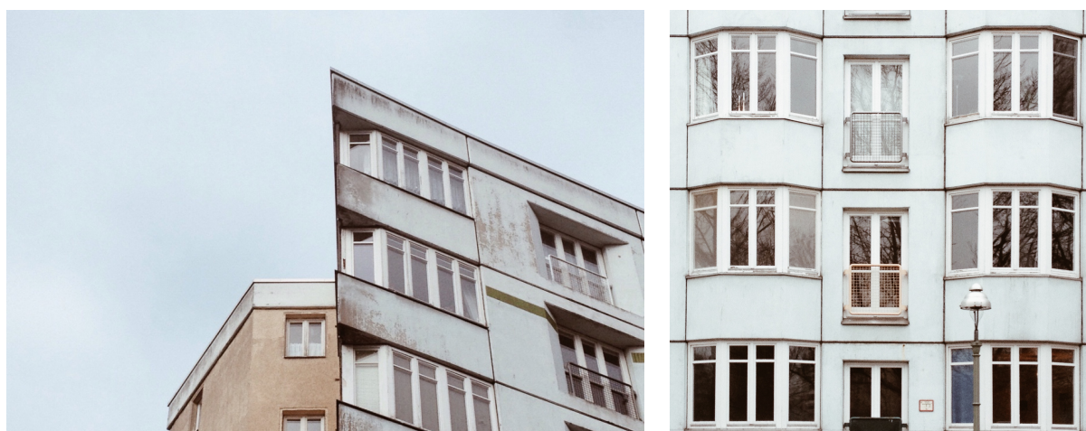
Figure 1: Housing Complex at Hansa Ufer 5 (photo by the author)
