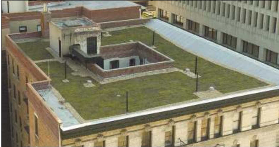
Green roof and research station site at 423 W. 118th Street
