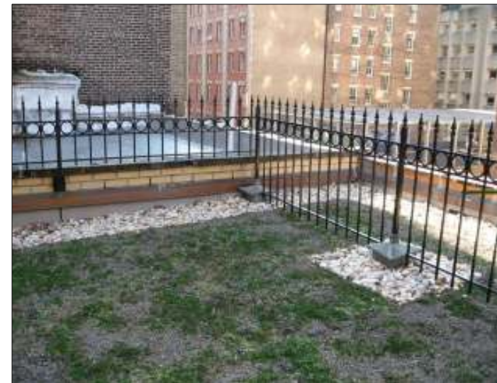
Green roof at 635 W. 115th Street
