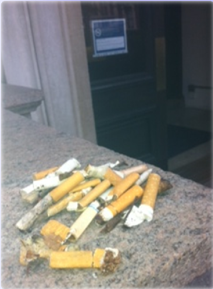
Mathematics Building. Prominent sign on east door. Butts within five feet of sign at entrance.
